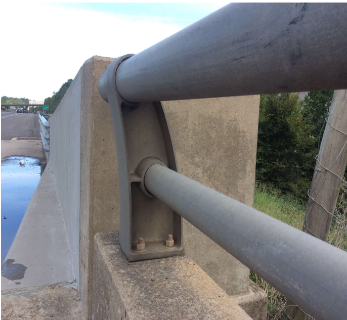
PHOTO 1 Description Loose bridge railing.
